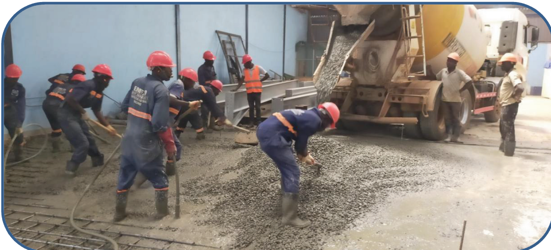
READY-MIX CONCRETE CASTING PROCESS FOR THE PROJECT
