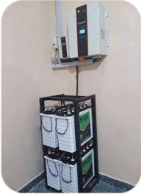
INSTALLED 1 ST & 2 ND FLOOR OFFICE INVERTERS
