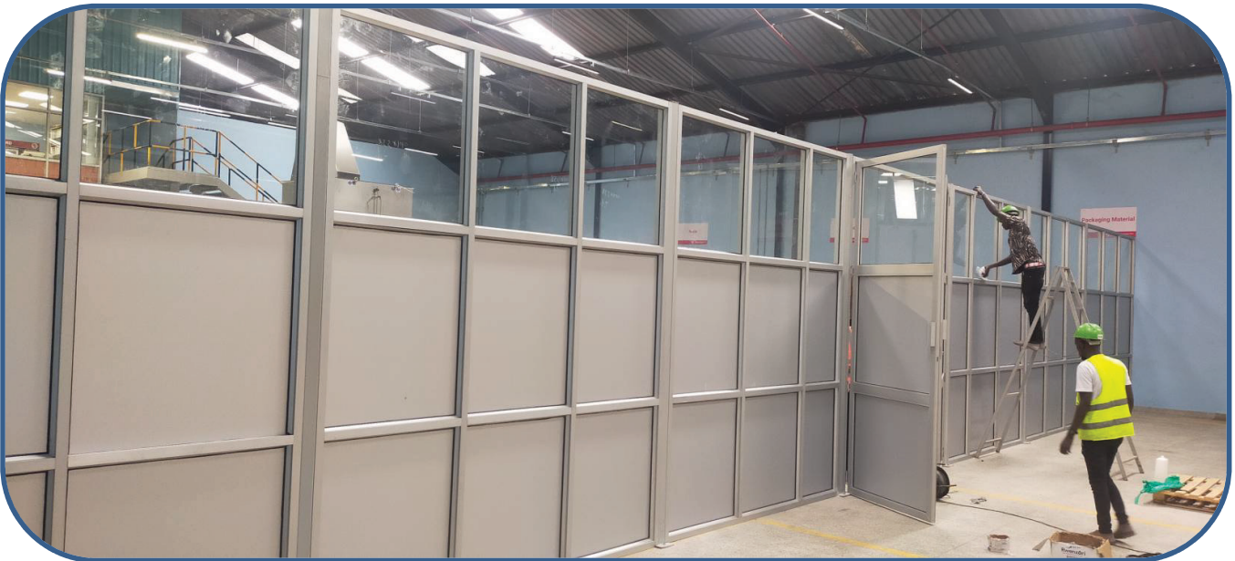
577 SQM ALUMINIUM PARTITION WALLS INSTALLED AT CCBU - RWENZORI PLANT
