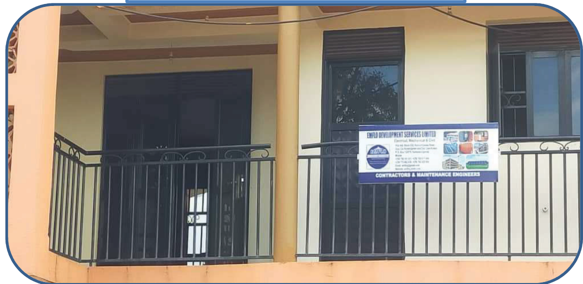
COMPANY OFFICE REAR SIDE VIEW
