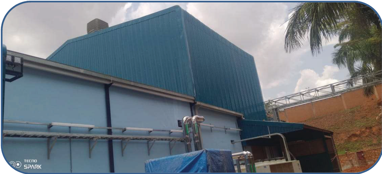
COMPLETED STRUCTURE OF PREFOM & CLOSURE MANUFACTURING PROJECT AT CCBU - RBC
